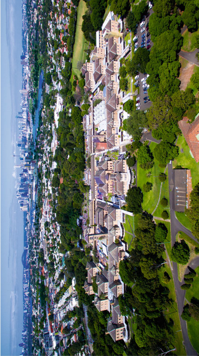
Fig. 13.1 Callan Park showing the Kirkbride Complex and proximity to Sydney, the Harbour Bridge and tip of the Opera House, February 2016 (Photographer: Jason Burcher; Retoucher: Thomas Ulman)
